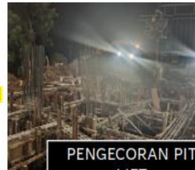
PENGECORAN PIT LIFT
