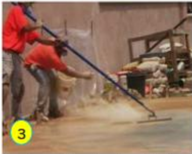
Penaburan Floor Hardener / Beton Trowel Finished
