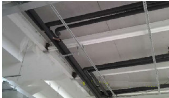
Percobaan Pipa Refrigerant
